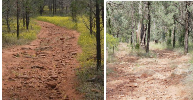
Figure 29 – Drainage and erosion issues
