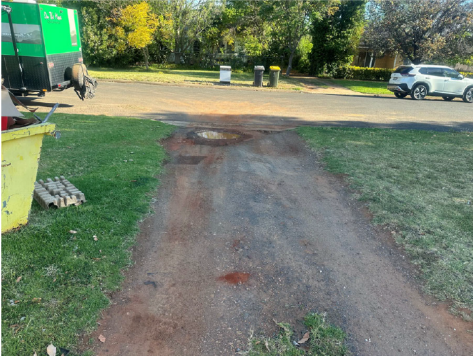
Existing layback and driveway – view to Hillston Road
