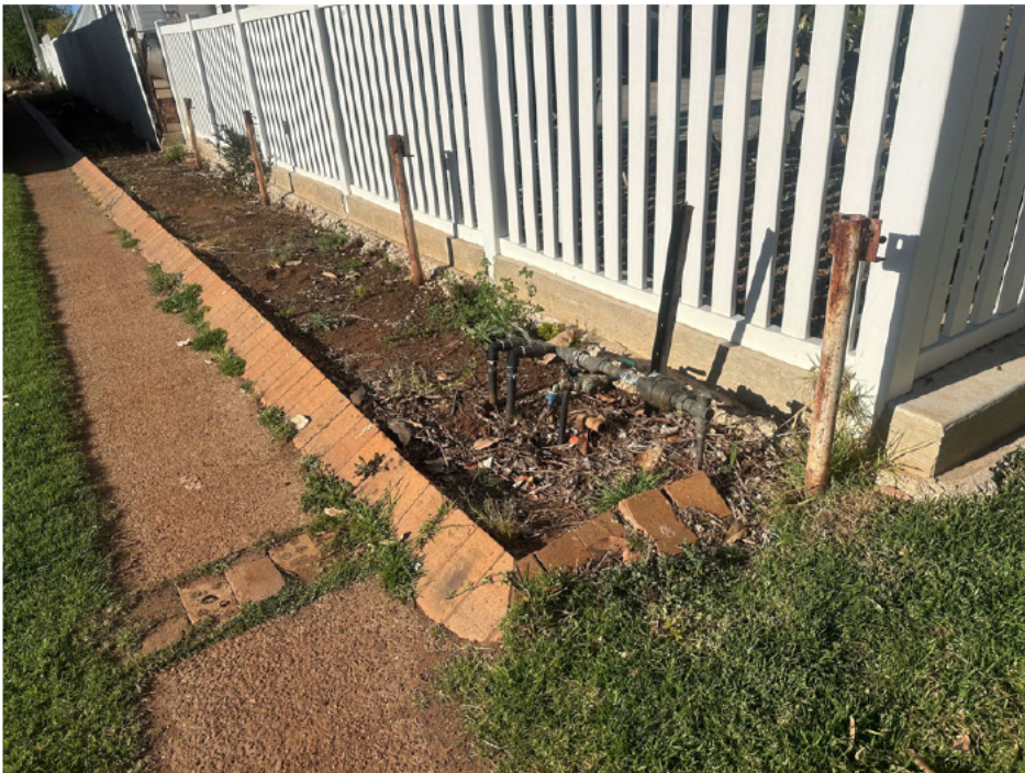
Eastern boundary front corner of site – water meter
