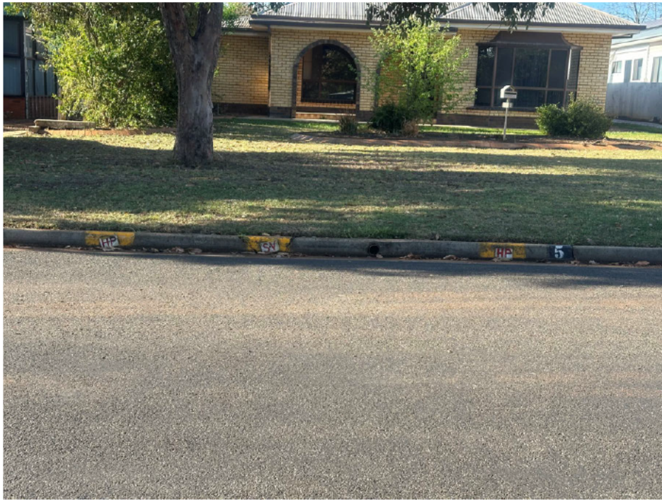
Frontage of site – note drain in gutter
