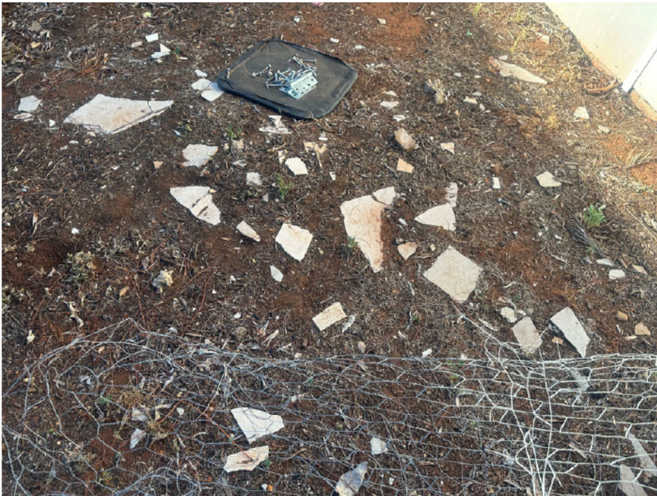
Broken fibro on north western corner of site. This will need to be removed during demolition and validation report provided.
