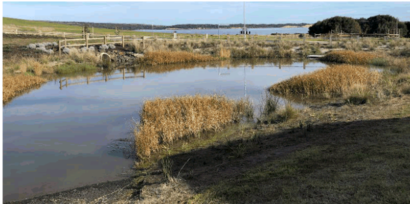
Figure 2 Typical Form of a Sediment Pond (San Remo Sediment Pond Designed by SWS in 2017)
