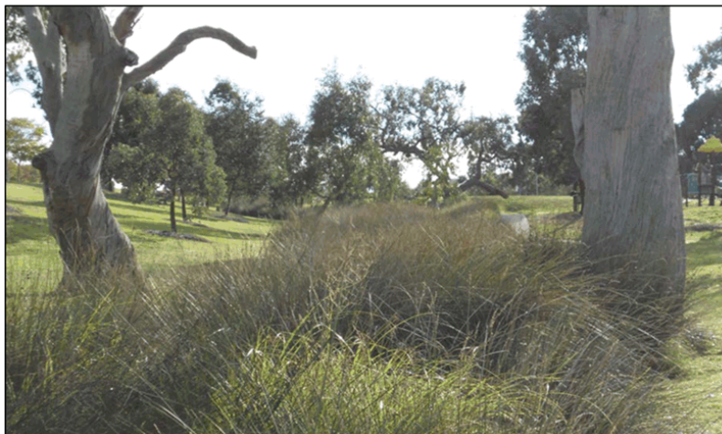
Figure 2 Typical Form of a Vegetated Swale in a Parkland Setting (Photo SWS 2018)
