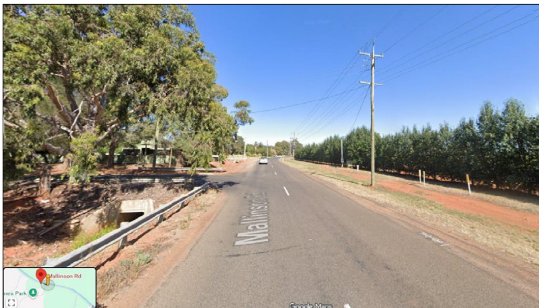
Figure 4: Mallinson Road, view westbound on approach to the intersection with Maegraith Place (Source: Google Street View, Nov 2020)
