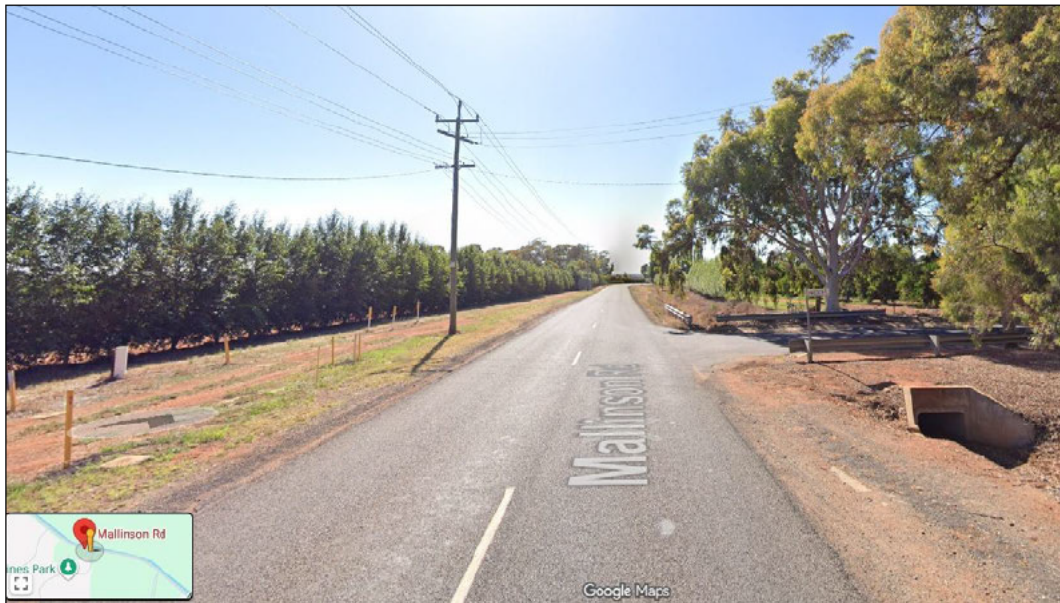
Figure 3: Mallinson Road, view eastbound on approach to the intersection with Maegraith Place (Source: Google Street View, Nov 2020)
