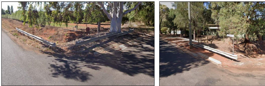
Figures 16 & 17: Existing guard fence installations at Maeграith Place intersection (Google Streetview).
