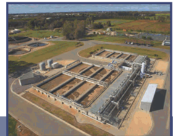
Water Reclamation Plant membrane replacement
