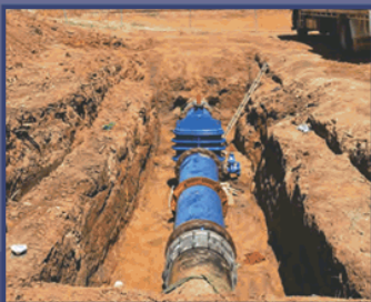
New Sewer Rising Mains (G2 to G1 Sewer Pump Stations)
