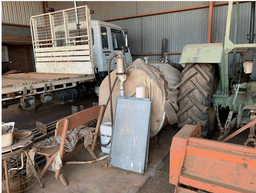
Photograph 5: Above ground disused fuel tank inside the machinery shed.
