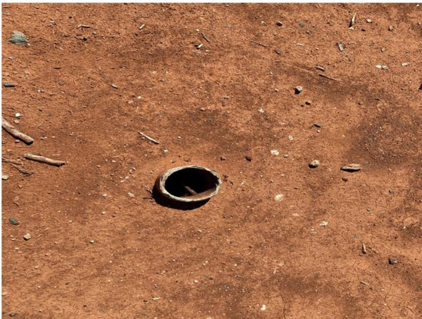
Photograph 2: Tile drainage with asbestos riser.
