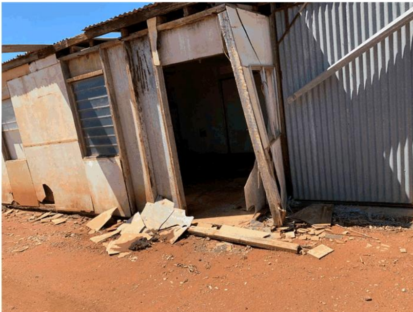
Photograph 10: Asbestos clad office attached to the packing shed, facing south. Broken ACM can be seen.
