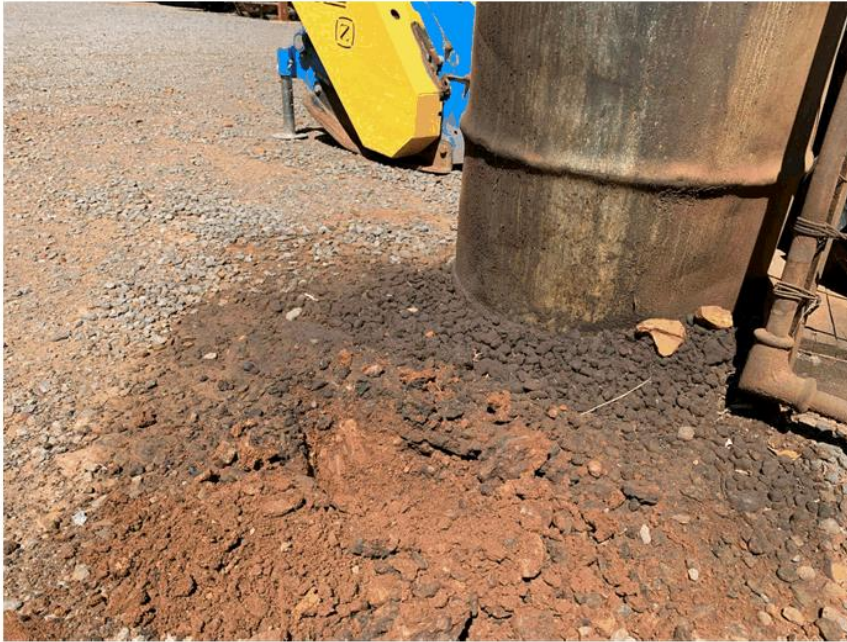
Photograph 7: Minor surface staining beneath the above ground fuel tank.
