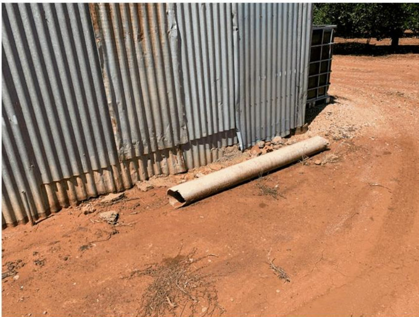
Photograph 2: Tile drainage pipe at the rear of the packing shed.
