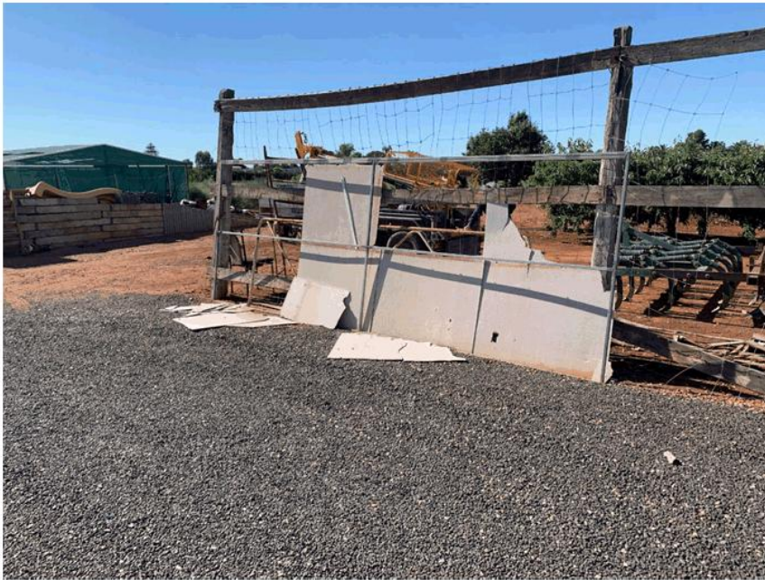
Photograph 13: Broken fibrous sheeting to the south of the greenhouse, facing north east.
