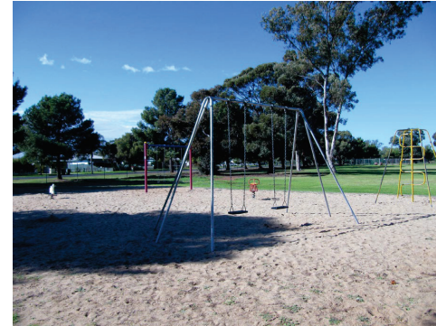
Figure 23: Aging Infrastructure (West End Oval)
