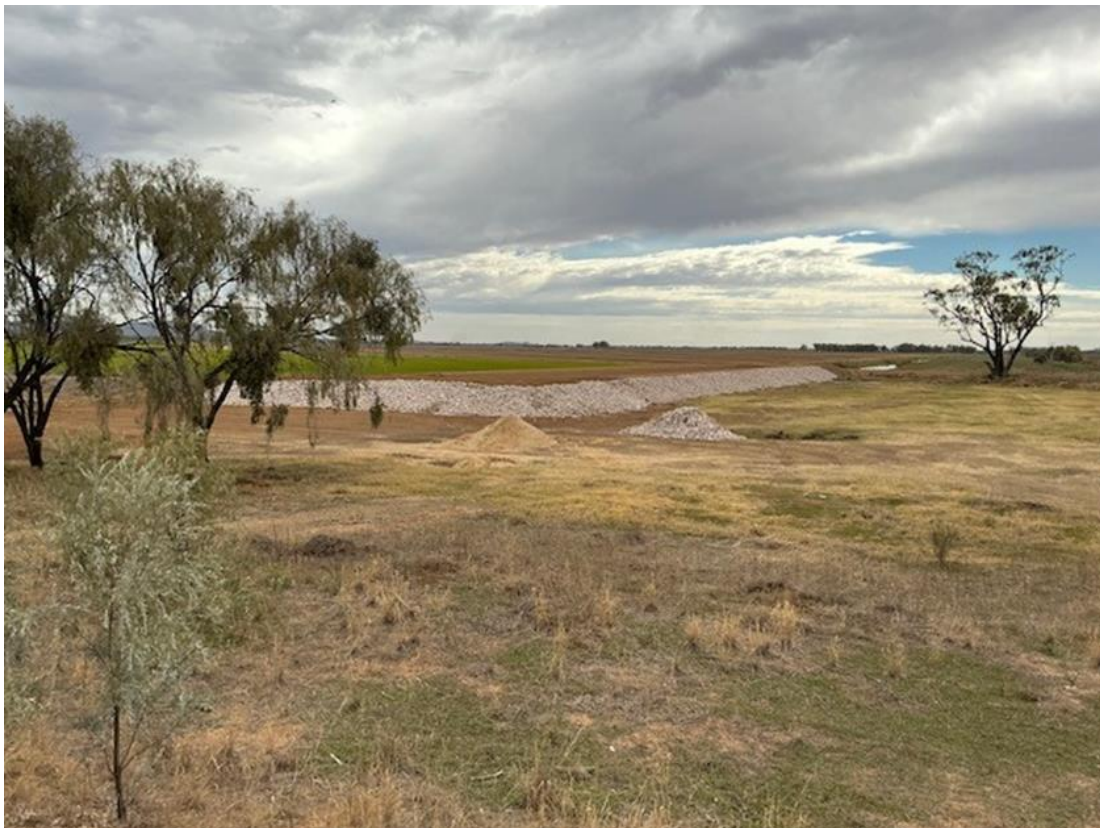
Photo looking North along the existing floodway on the Halse property. On the left is the bank protection provided by the MI North Merribee Channel Realignment. Photo taken 28 th February 2025.
