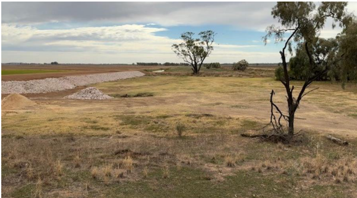
Photo looking North along the existing floodway on the Halse property. On the left is the bank protection provided by the MI North Merribee Channel Realignment.
