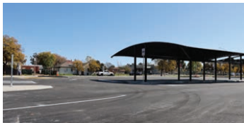
Railway Street car parks west and east completed.
