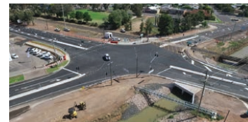
Yoogali Culvert Upgrade.
