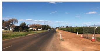
Collina Infrastructure works at Citrus Road/ Rifle Range Road.
