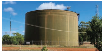
Griffith Water Reservoir (Scenic Hill) Refurbishment.
