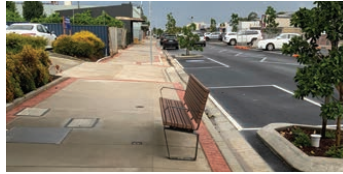
Yambil Street Stages 3 and 4 completed.
