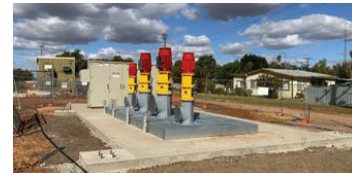
Hanwood Flood Pump and levee project - underway.
