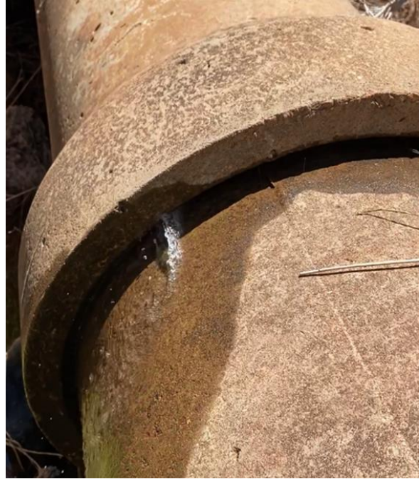
Photo 2 – Leakage at the concrete pipe joint
