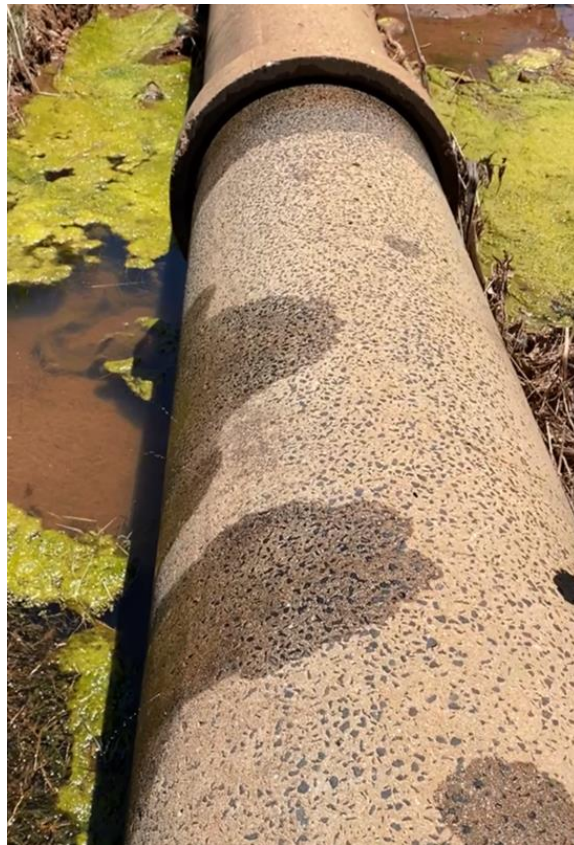
Photo 3 – Leakage along the concrete pipe
